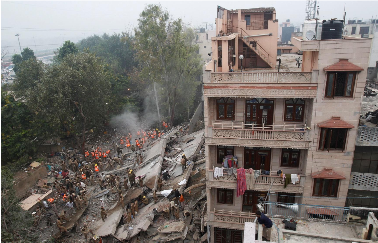
The Lalita Park building collapse 15 November 2010 in the Indian capital of New Delhi . 66 dead and 80 injured
